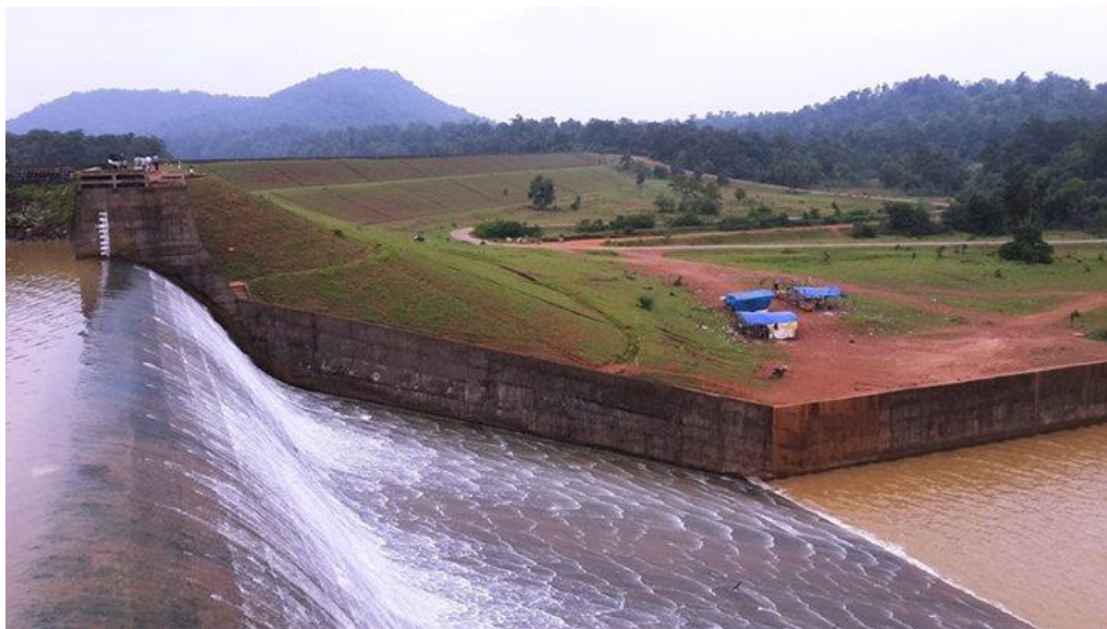
Fig. 3.6 Pictorial view of Spillway of Paralkot dam
